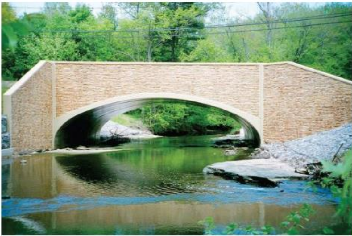
Figure 7.3 - Bottomless culvert (7-6)
