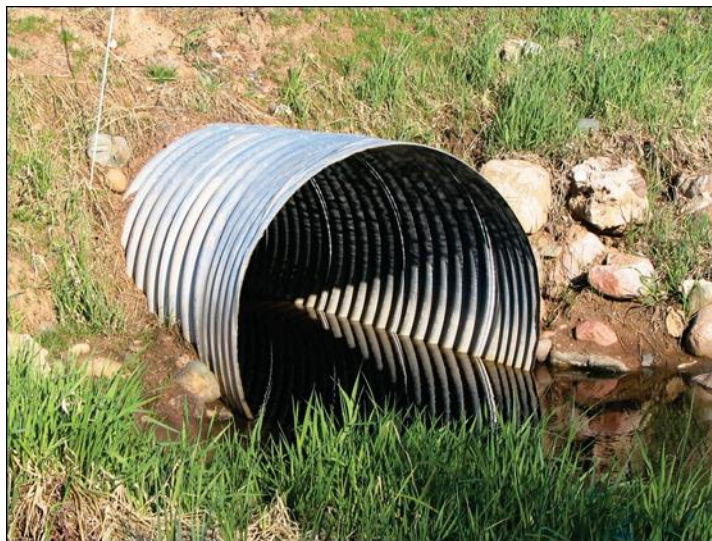
Figure 7.11 Corrugated metal pipe (7-6)
