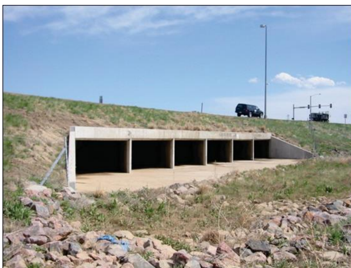
Figure 7.12 Multiple barrel box culvert (7-6)
