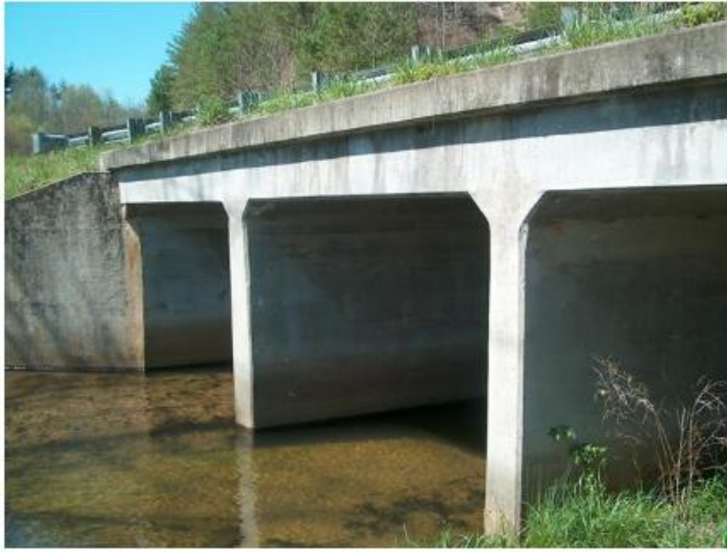
Figure 7.4 - Embedded box culvert
