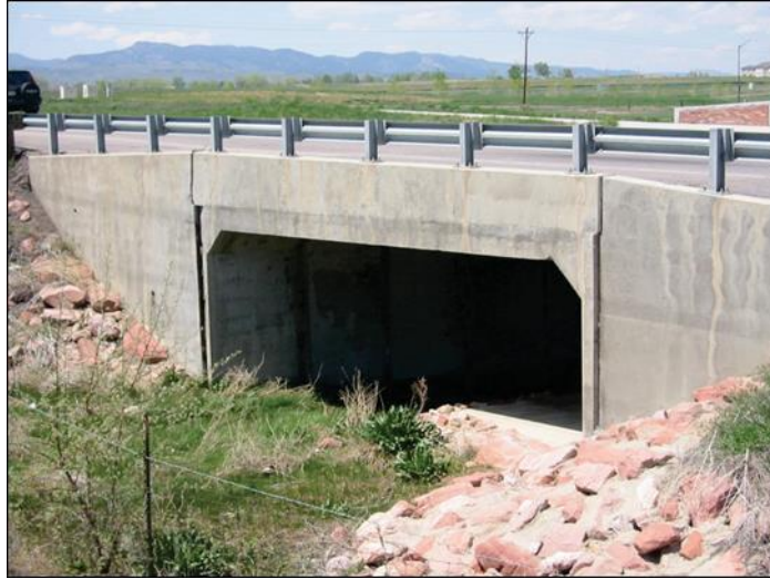
Figure 7.10 Concrete box culvert (7-6)
